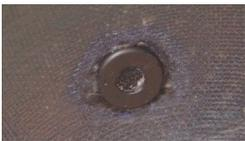
7. Ensure the Valve Base fits flush with the inside of the socket.
