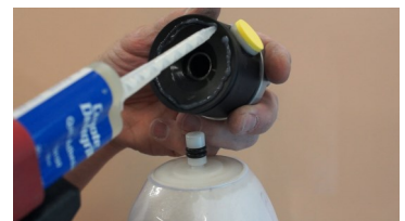
Pull a PVA bag over the anchor and cast. Glue your lock to anchor and start laminating.
